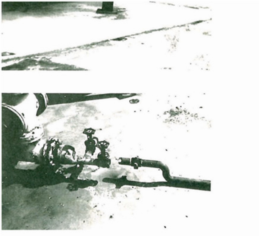
Figure B.8. Detail of the rupture of a pipe by the attached tank sliding in an oil field near Coalinga
