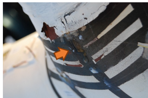
(d) Crack penetration at a wall thinning tee (Tee2 of AP3_EC01, NIED_Test#03)
